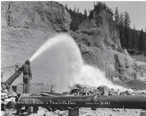
Vintage photo of hydraulic mining in California showing a water cannon or monitor (also referred to as a "Giant" and hill side of alluvial material being washed with the gold ultimately being collected in a sluice box or "long tom".
