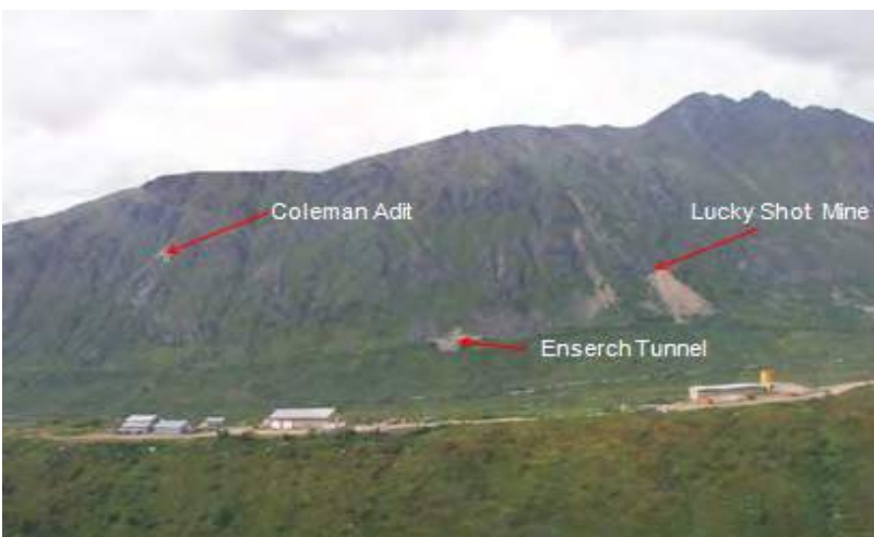
Willow Creek project today with the Coleman, Lucky Shot and Enserch tunnel which could provide valley access to the Coleman mineralization as well as providing underground drill stations for future exploration.
