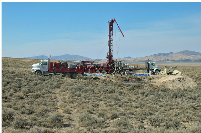
Drill testing at Red Hill northwest of drill intercept BRH-013
