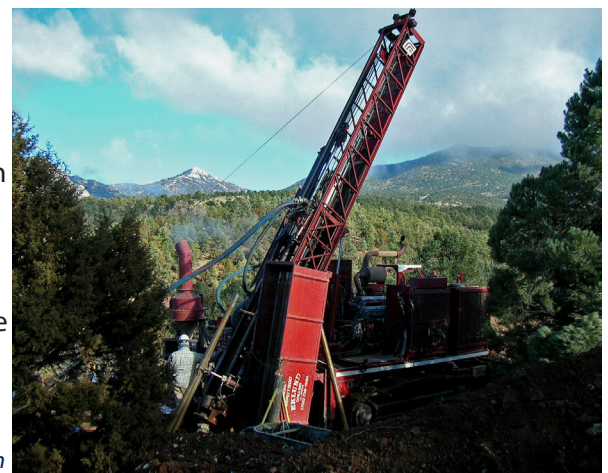
Drilling at Red Canyon
